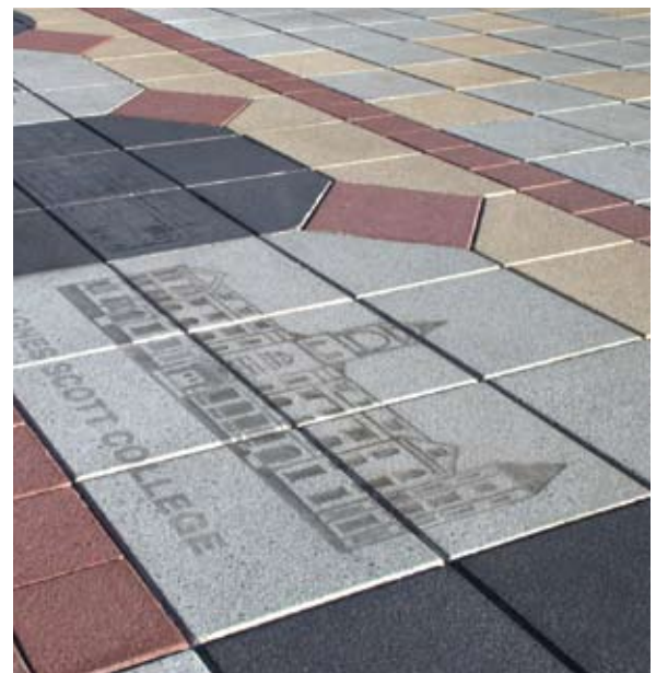
Graphics etched in the paving slabs from water jet techniques depict Decatur landmarks and history.
